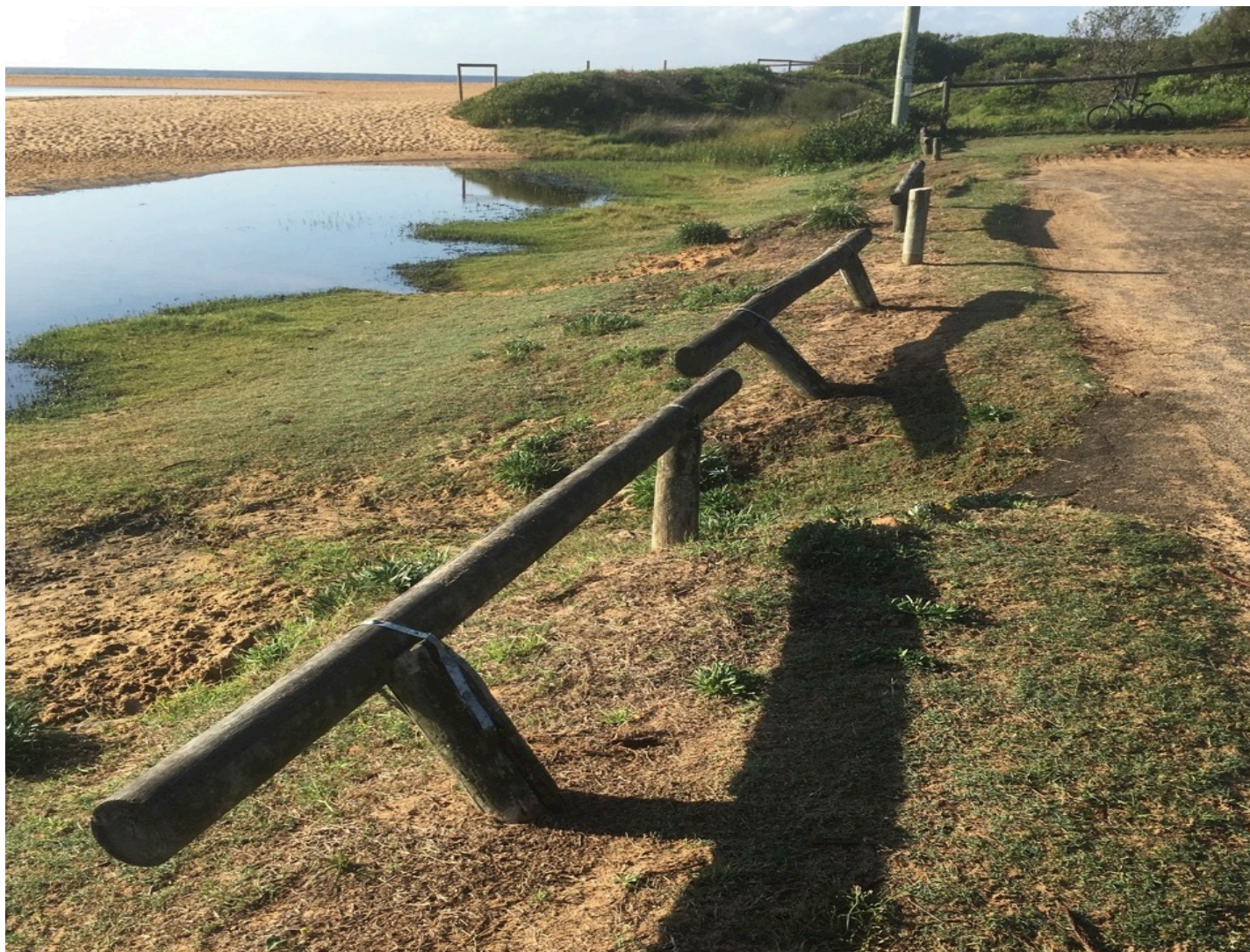
Figure 6: The poor state of log barriers – Lagoon foreshore.
